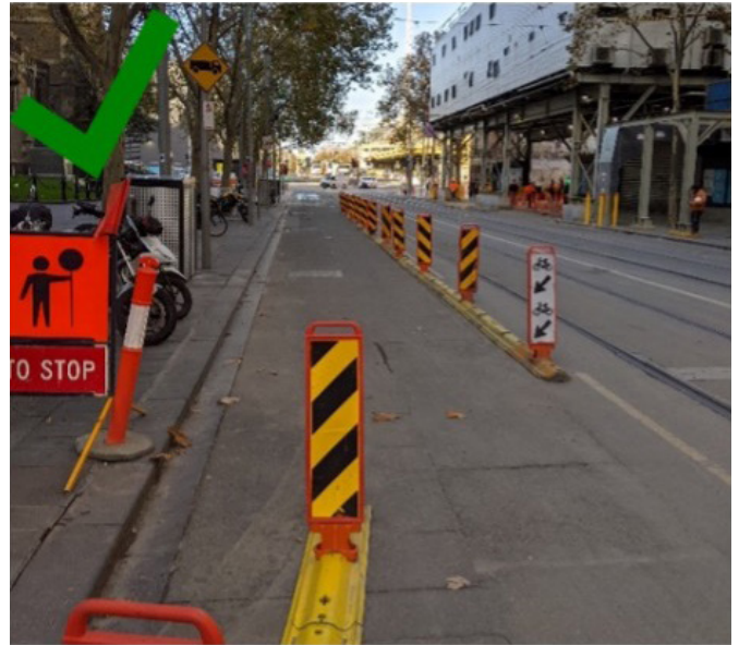
Figure 3. Temporary barriers to protect cyclists from truck movements out of site
