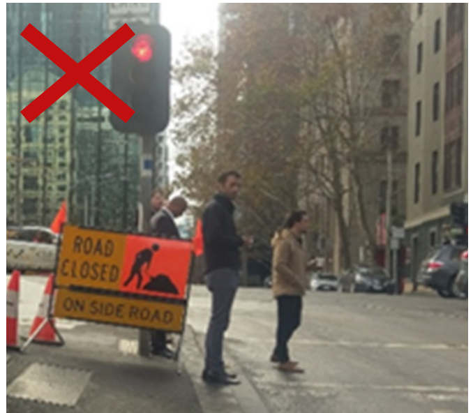
Figure 4. Temporary sign leaving inadequate width on footpath for pedestrians
