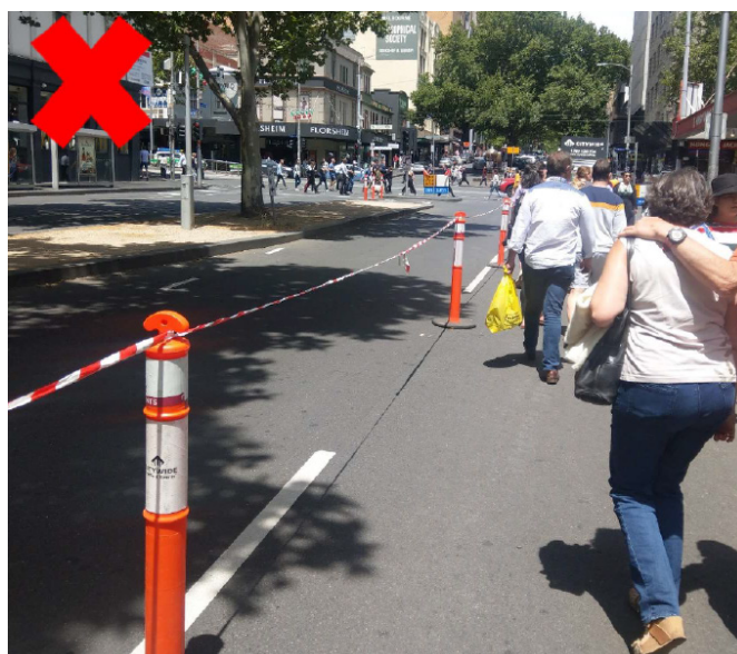
Figure 2. Incorrect usage of tape adjacent to live traffic lane
