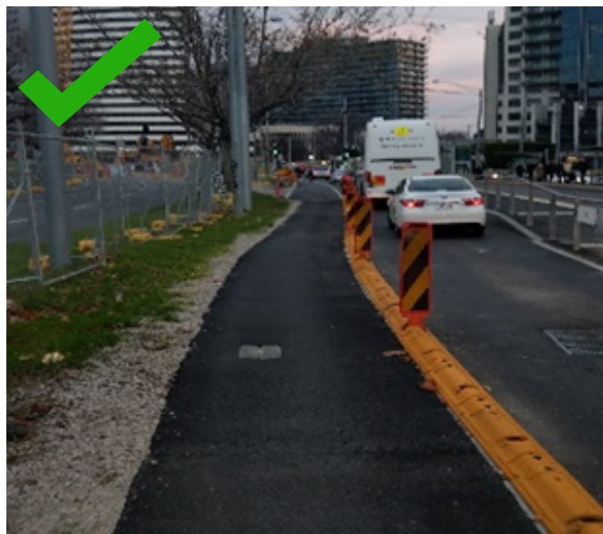
Figure 1. Delineation of cyclists from traffic lane
